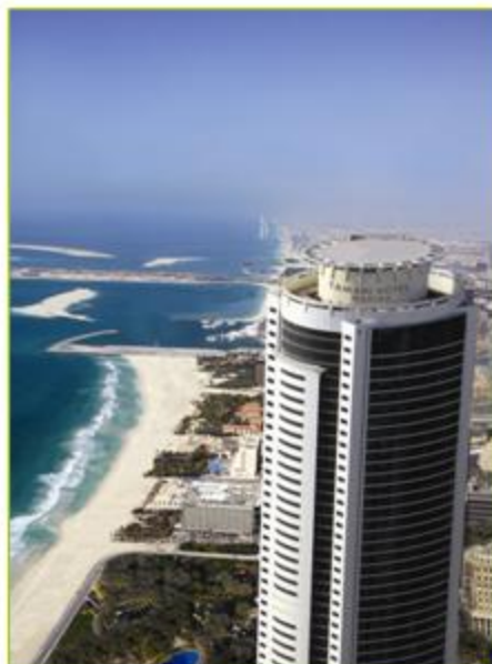
TAMANI Hotel Marina tower overlooking The Palm Island, Jumeirah
